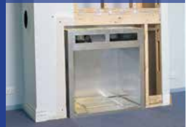
Heater fitted to Zero Clearance Box
