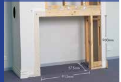
Zero Clearance Box positioned in framework
