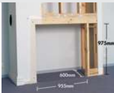
Timber framework, partially plaster board cladded
